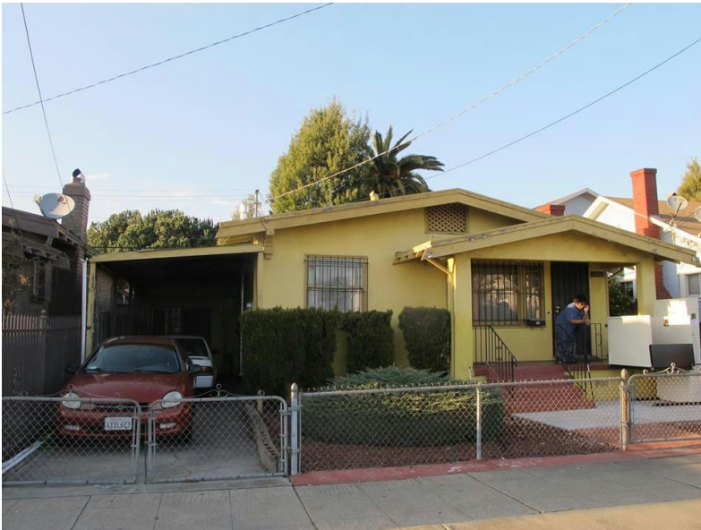
Above: Workplace for this April's RTO project
